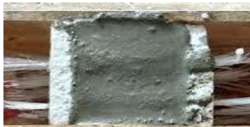
Figure-7: Concrete placing in mould
