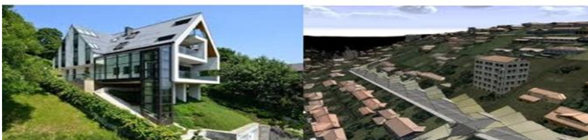
Figure-1: Buildings on sloping ground
